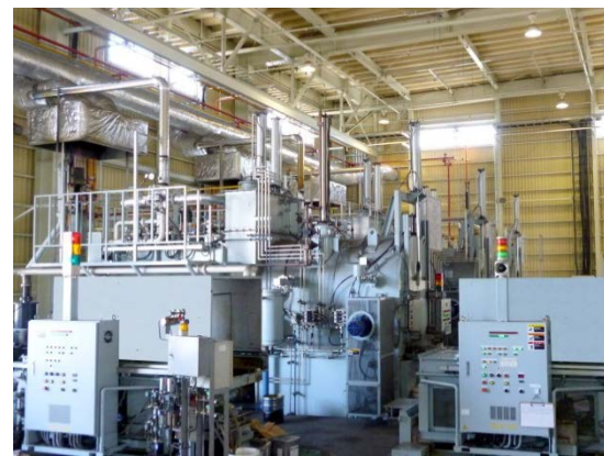
Heat processing equipment
